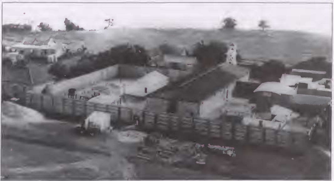
Fig. 4. 1930s aerial photograph of the Gaol. Area A tank is visible beyond the white kitchen building, in the top left (southwest) corner of the area enclosed by the perimeter fence. Note also the above-ground water tank on a stand in the lower left (southeast) corner of the Gaol, in front of the infirmary. (Photo: Museum and Art Gallery of the Northern Territory).
